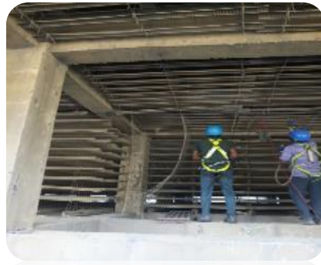
Cooling Tower Overhauling
