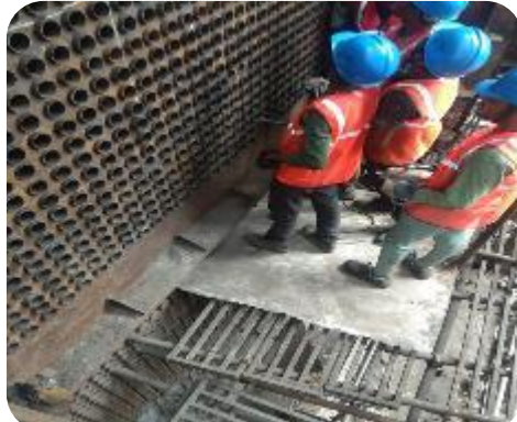
APH Tube Replacement
